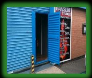
Outside opening gates, are designed to allow the gate and the outer frame to open outwards. This type is predominantly used when the shutter is fixed to the outside of the building.
