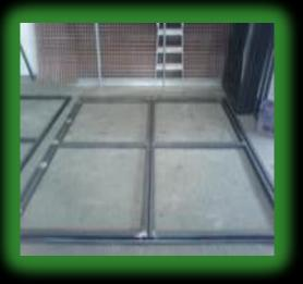
British made from: 40mm x 40mm or 25mm x 25mm box section fully welded for maximum strength.
